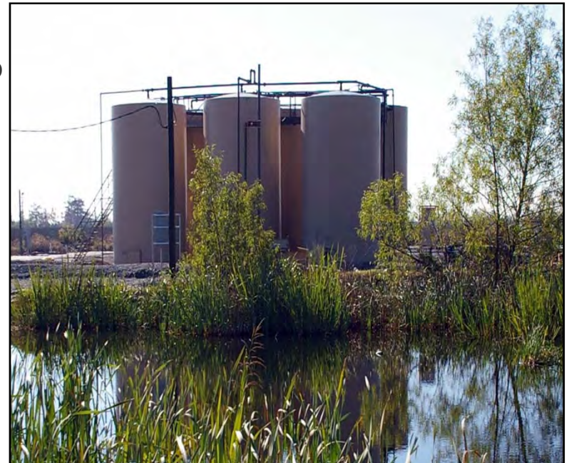
East Chalkley Tank Battery
